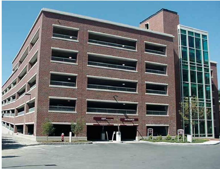
275 Grove Street Garage.
