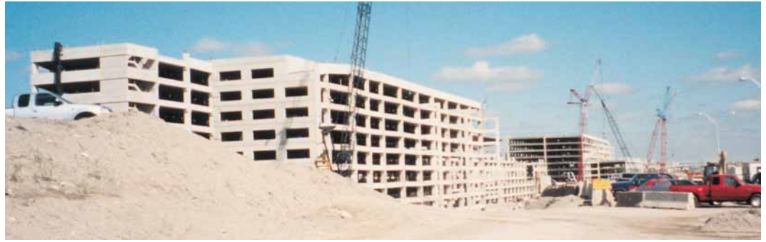
7 cranes at work on the Midfield Terminal Parking Garage.
