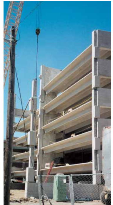
401 Water Street garage nearing completion.
