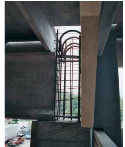
Girder to column connection prior to cast-in-place pour.
